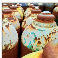
Rusty / Fatigued Cylinders
